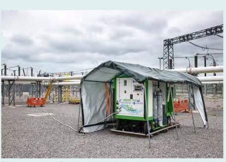
Onsite gas cart used to retro fill existing gas-insulated, high-voltage switchgear, with an alternative low global warming g<sup>3</sup> gas, designed for high-voltage transmission equipment, Richborough Substation, Kent, UK
